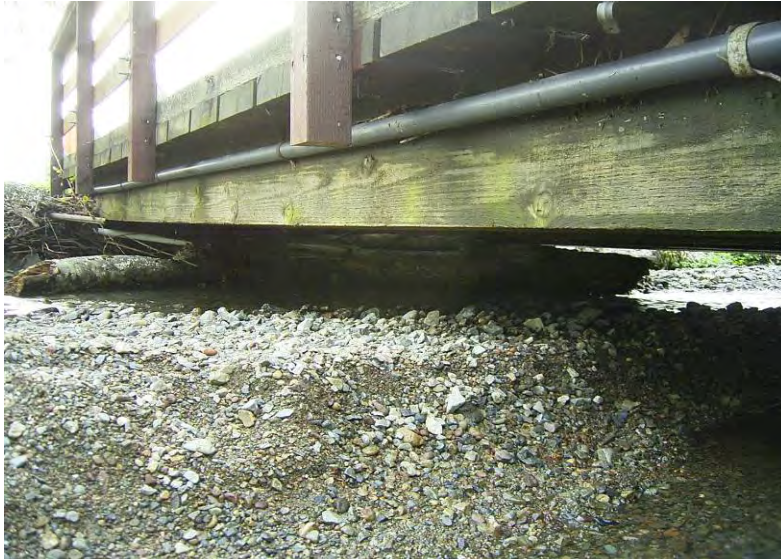
Figure 4 - Bridge crossings over Easkoot Creek.
