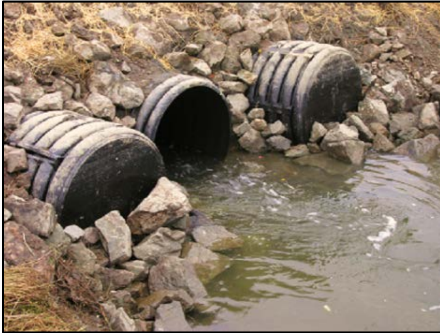
New McAllister Slough Culverts with 2 pipes capped off for future use
